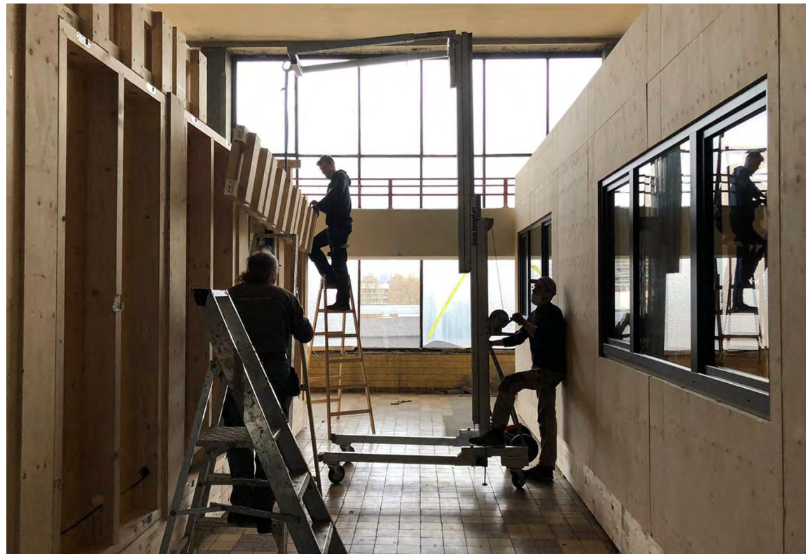
[Fig. 24] WBX Pilot project at Molenbeek construction site Source: Vitor Breder
