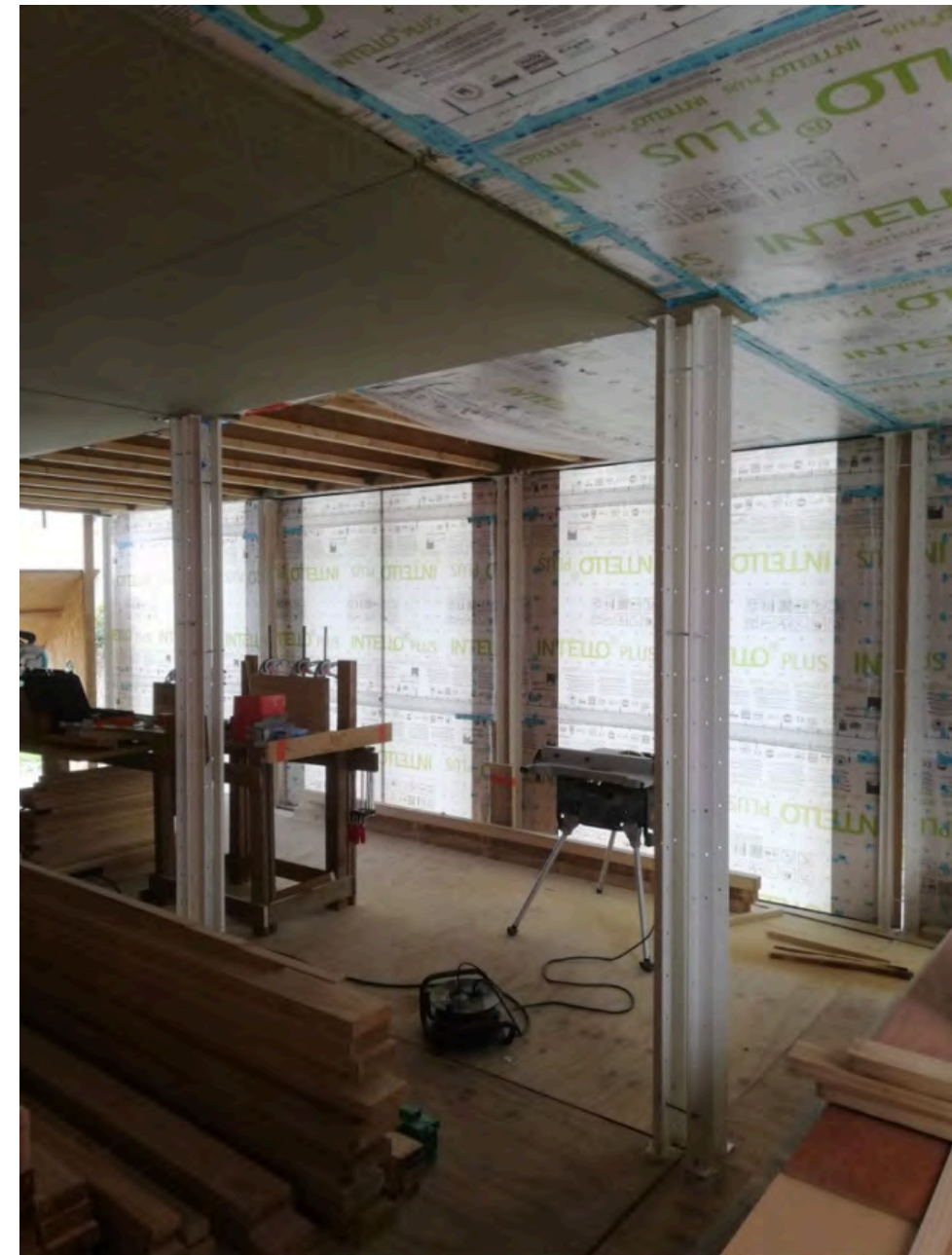
[Fig. 21] SMH Pilot project at Jette interior view Source: Alt_Shift* Archive
